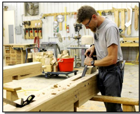
Hand work on joinery assures accuracy
