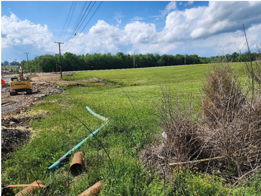
Subject property primary frontage, photograph taken facing westerly
