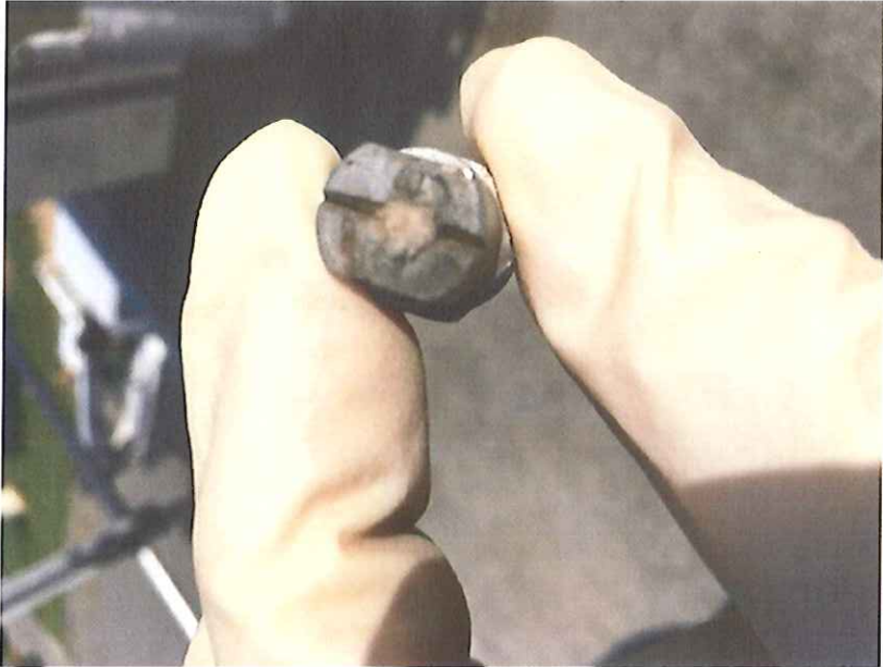
Clogged spray head.
