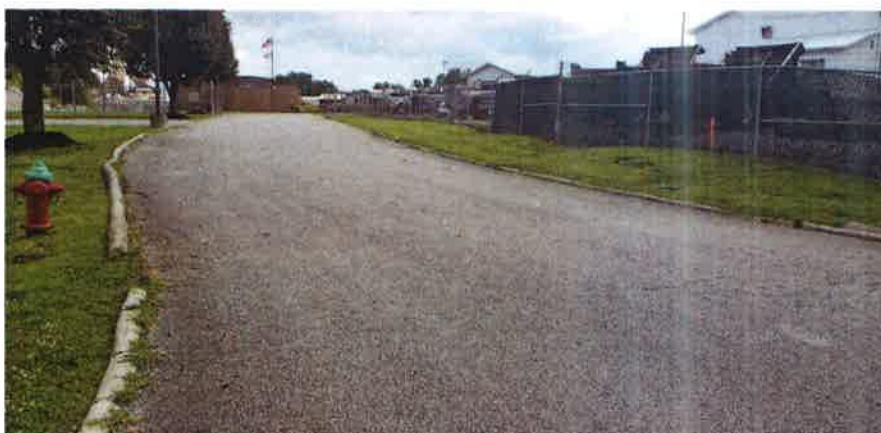
DATE TAKEN: 7/20/2021 VIEW NORTH STR. 3 DRIVEWAY, STR. 1 FENCE & STR. 2 GRAVEL PARKING AT RIGHT
