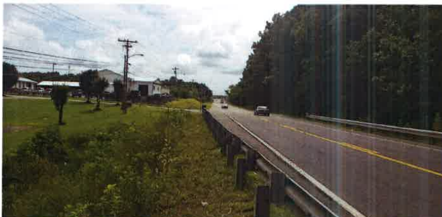
DATE TAKEN: 7- 7/20/2021 VIEW EAST FROM PROPOSED BRIDGE REPLACEMENT ALONG SPARTA HIGHWAY & TRACT 24 AT LEFT
