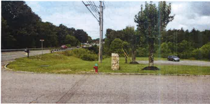
DATE TAKEN: 7/20/2021 VIEW WEST ALONG SPARTA HIGHWAY, PROPOSED FEE ACQUISITION AND PROPOSED BRIDGE REPLACEMENT FROM DRIVEWAY (STR. 3) ON TRACT 24
