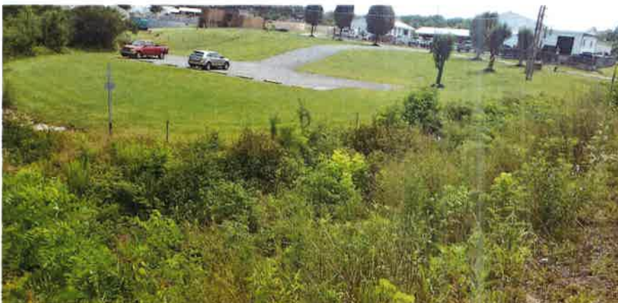
DATE TAKEN: 7/20/2021 VIEW NORTHEAST ACROSS WESTERN PROPOSED FEE ACQUISITION AREA & CITY OF CROSSVILLE SEWAGE FACILITY FROM PROPOSED BRIDGE REPLACEMENT & SPARTA HIGHWAY
